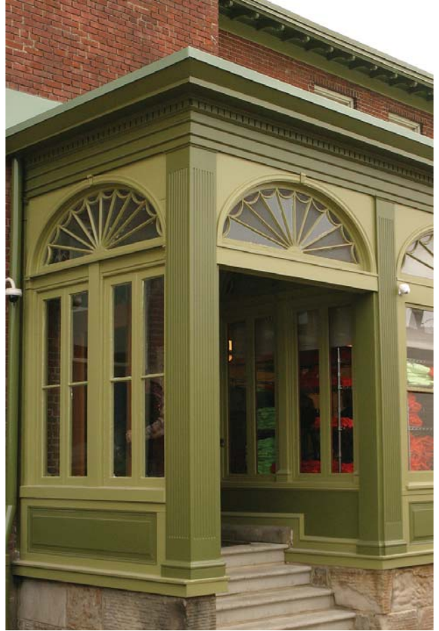
The side entrance, before and after.
