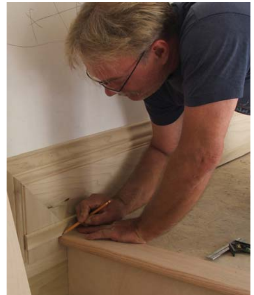
A carpenter finishes woodwork in the meeting room.
